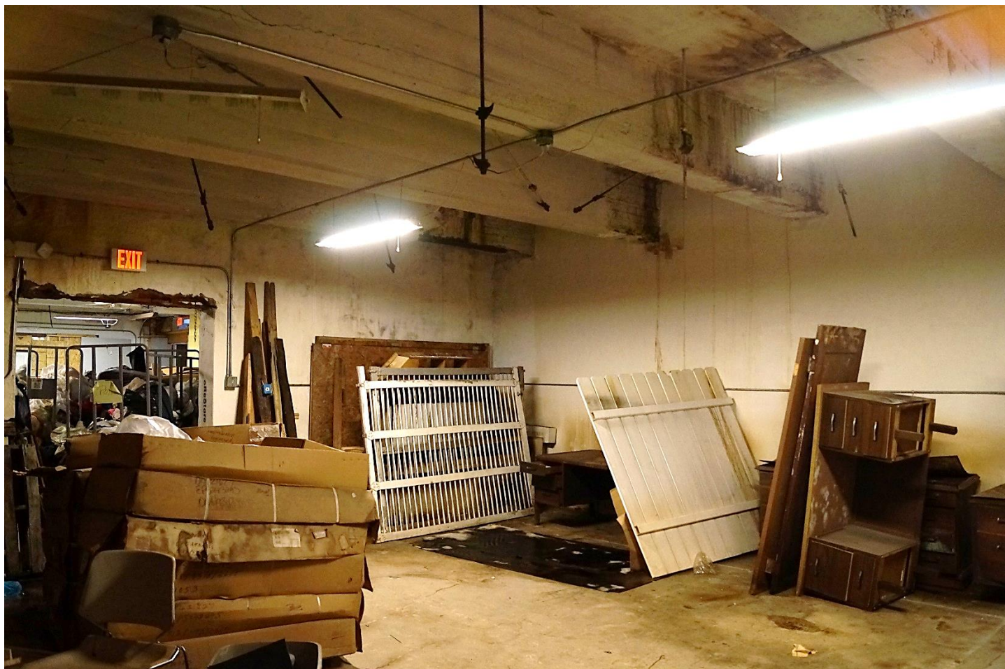
Photo 9: Interior of Deep Cold Storage Space, Isaacs & Sons Cold Storage Building. View South. Scott Wiczorek. July 26, 2023.
