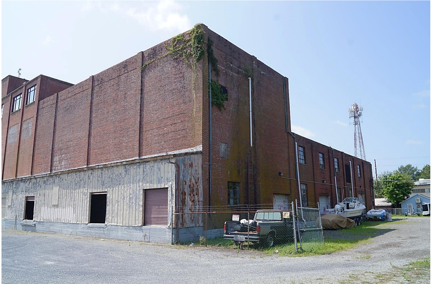
Photo 4: Isaacs & Sons Cold Storage Building. View South. Scott Wieczorek. July 26, 2023.
