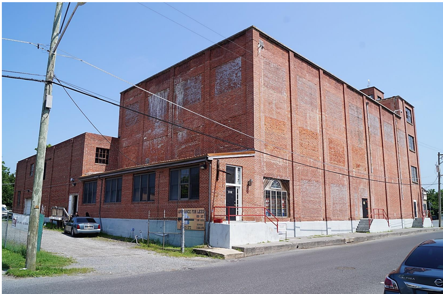
Photo 1: Isaacs & Sons Cold Storage Building. View North. Scott Wieczorek. July 26, 2023.
