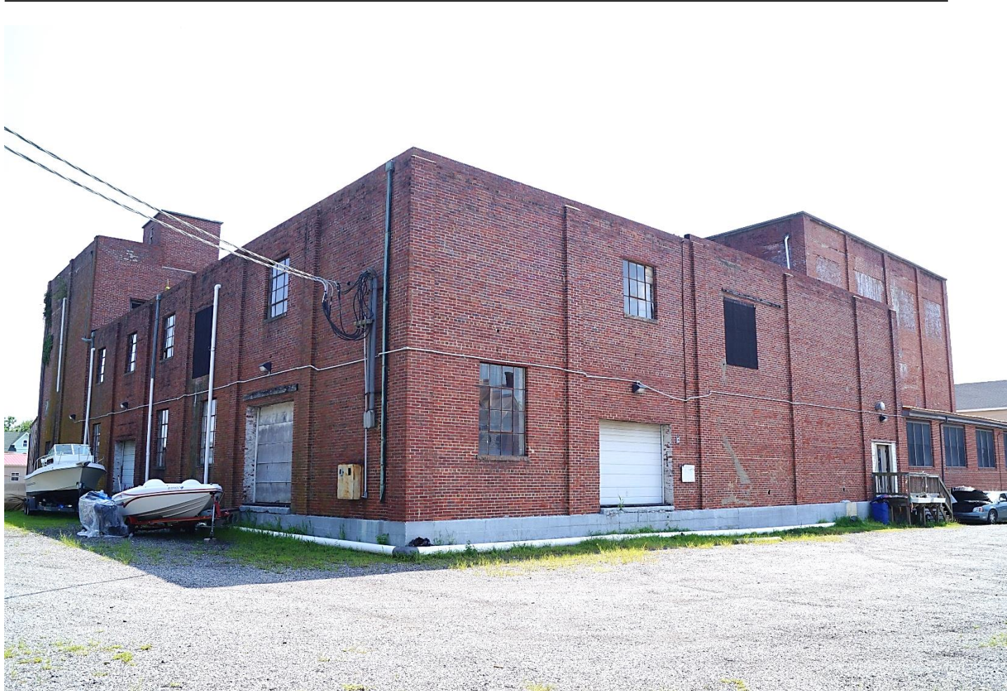
Photo 5: Isaacs & Sons Cold Storage Building. View East. Scott Wiczorek. July 26, 2023.
