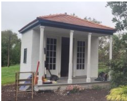
Excavation sheds light on Buena Vista building
