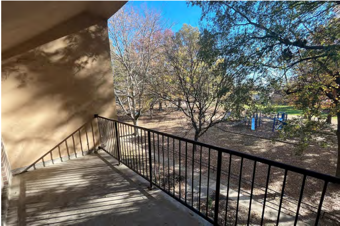
27. 620 N. Walnut St (Type B Typical): 3rd floor, apartment balcony, looking northeast.
