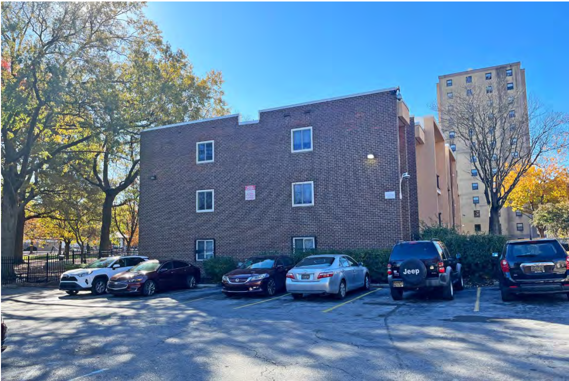
10. 630 N. Walnut St: north elevation, looking south.
