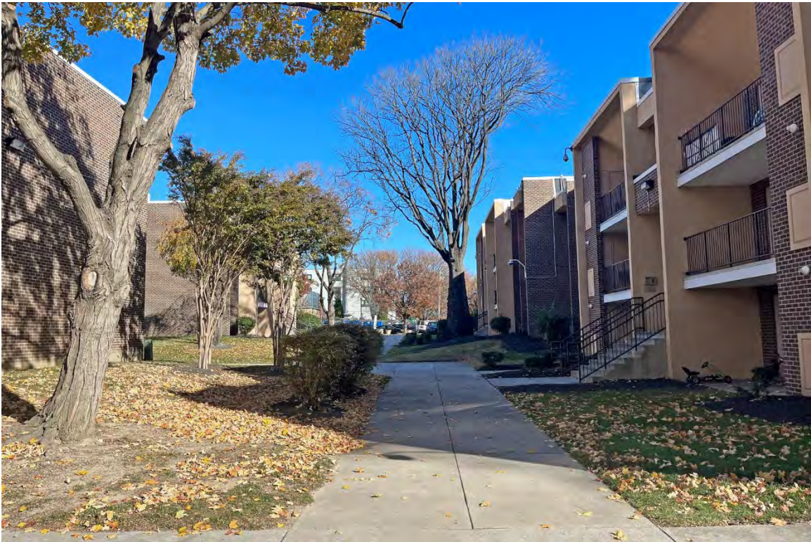
2. Central courtyard and walkway, looking north.
