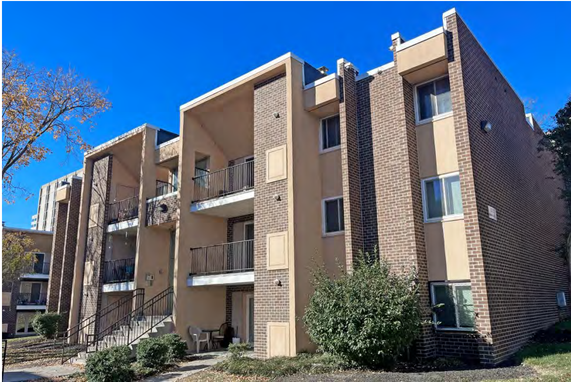
11. 640 N. Walnut St: east elevation, looking southwest.
