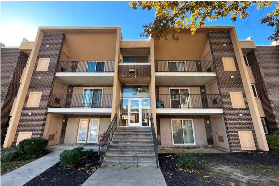
16. 650 N. Walnut St: north elevation, looking south.
