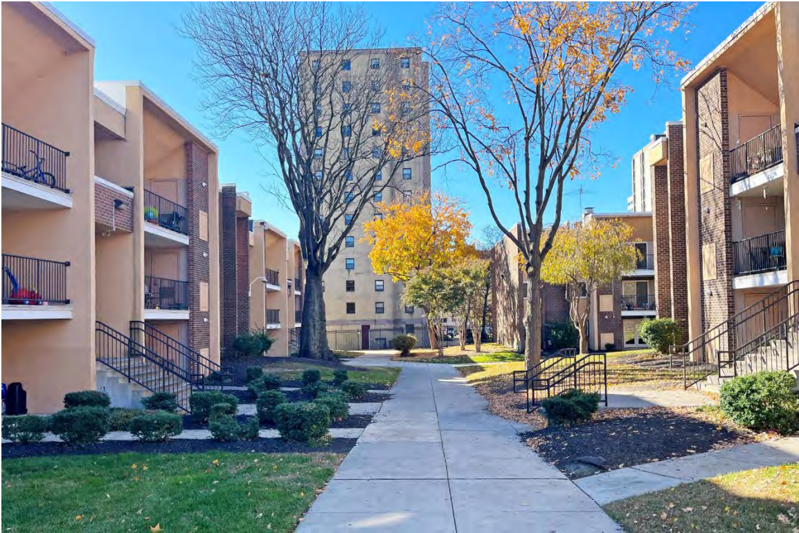
1. Central courtyard and walkway, looking south.
