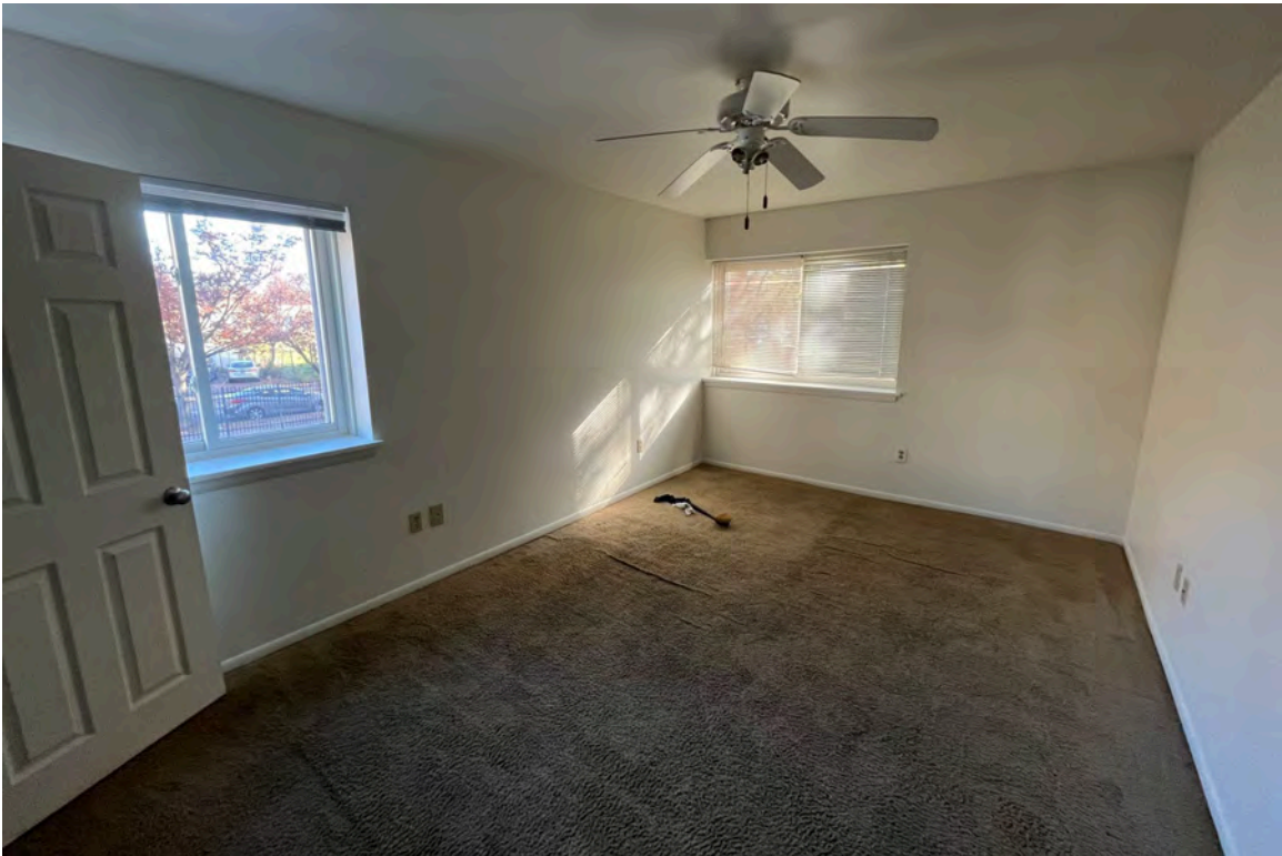
26. 650 N. Walnut St (Type B Typical): 3rd floor, apartment, looking southeast.
