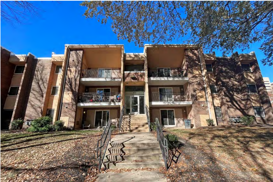
8. 630 N. Walnut St: east elevation, looking west.
