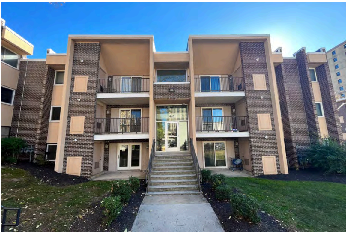
14. 640 N. Walnut St: west elevation, looking east.
