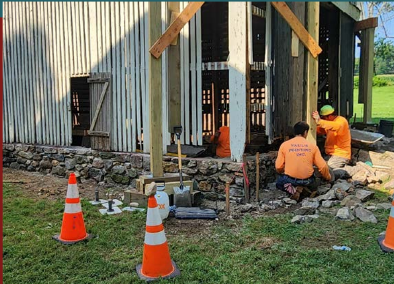
Foundation repair work on Granary at Cooch's Bridge
