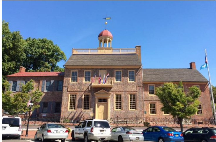
The roof of the New Castle Court House Museum was replaced in the spring of 2015.
