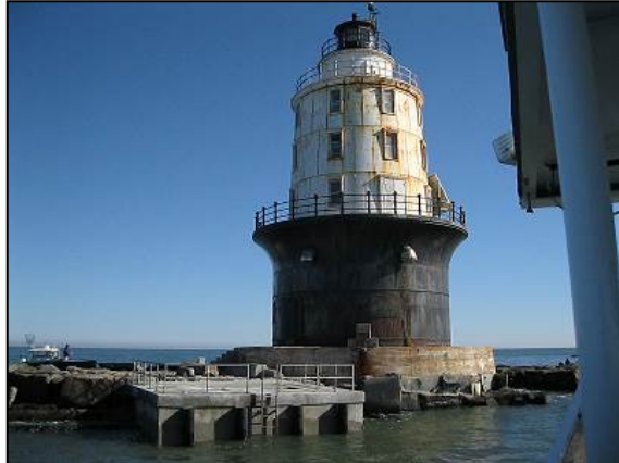
Remaining section of the Harbor of Refuge Lighthouse dock after damages caused by Hurricane Sandy (left), and the lighthouse with its new dock (right).
