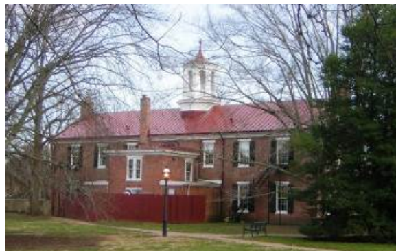
The Arsenal with newly painted and repaired cupola and roof.
