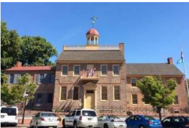
New Castle Court House Museum with new roof.
