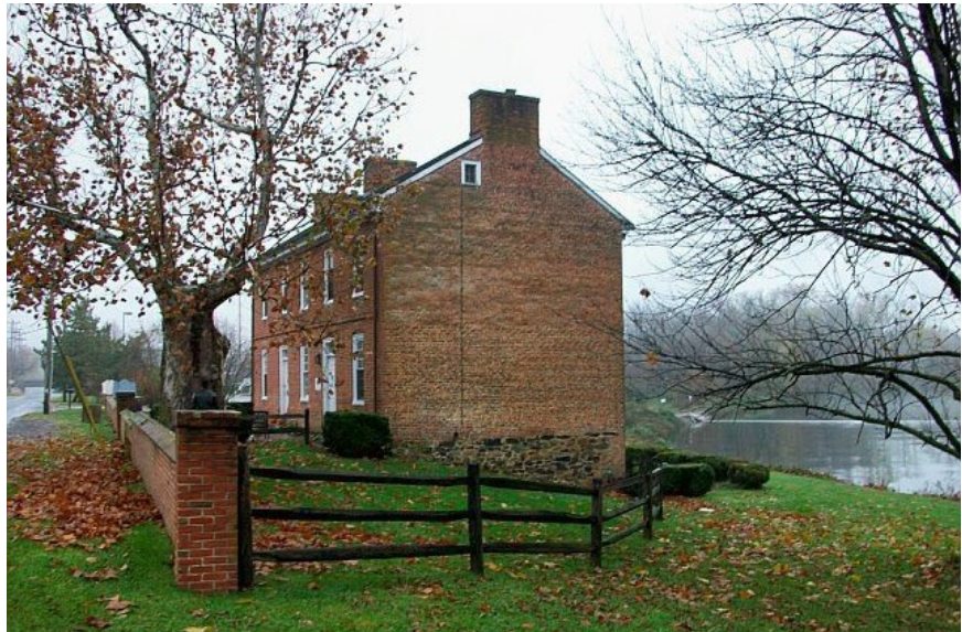
(Top) Deteriorating mortar joints at one of the gables of the Hale-Byrnes House. (Bottom) Exterior view of the historic home.
