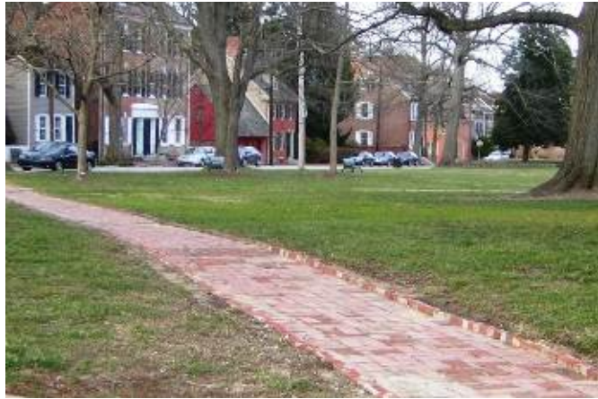
Repaired sidewalk on the New Castle Green.
