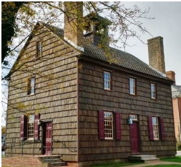
Photos of the Old Sussex County Court House before (top) and after restoration work.
