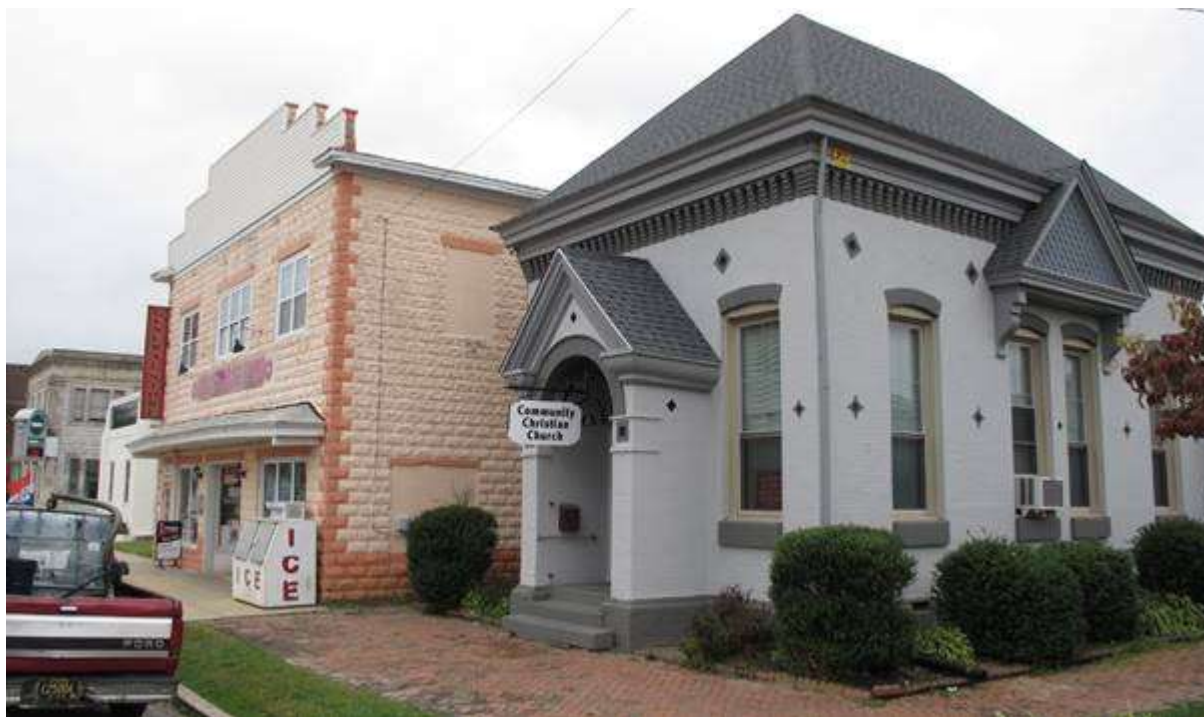
Commercial buildings along Commerce Street in Harrington
