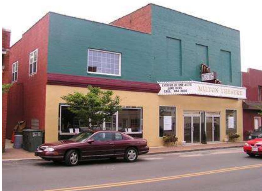
The Milton Theatre today. The building is a component of the Milton Historic District.
