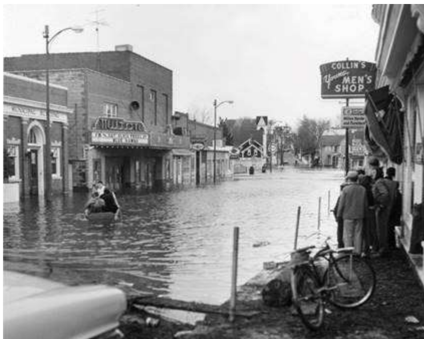
Flooding along Union Street in front of the Milton Theatre in Milton, Del. after the March 1962 nor'easter. Disaster preparedness for historic properties will be explored as part of the upcoming historic preservation symposium.
